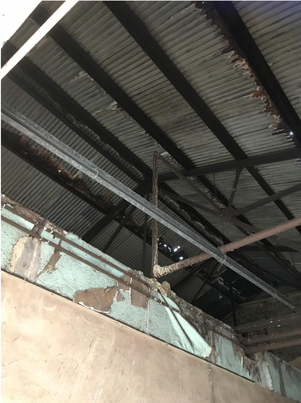
Photograph 10 – Interior of welfare block of structure B1b, note poor condition of corrugated metal roof
