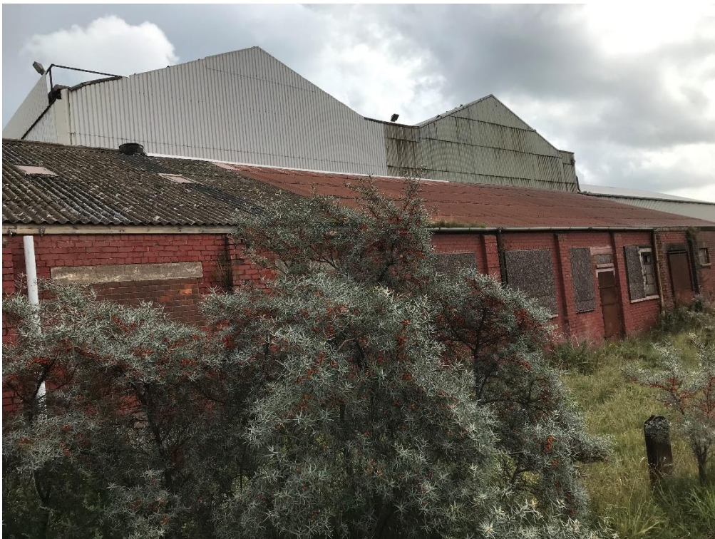
Photograph 6 – South-western elevation of structure B1b, welfare block with corrugated metal roof and boarding windows to the right, canteen block with corrugated asbestos roof to the left
