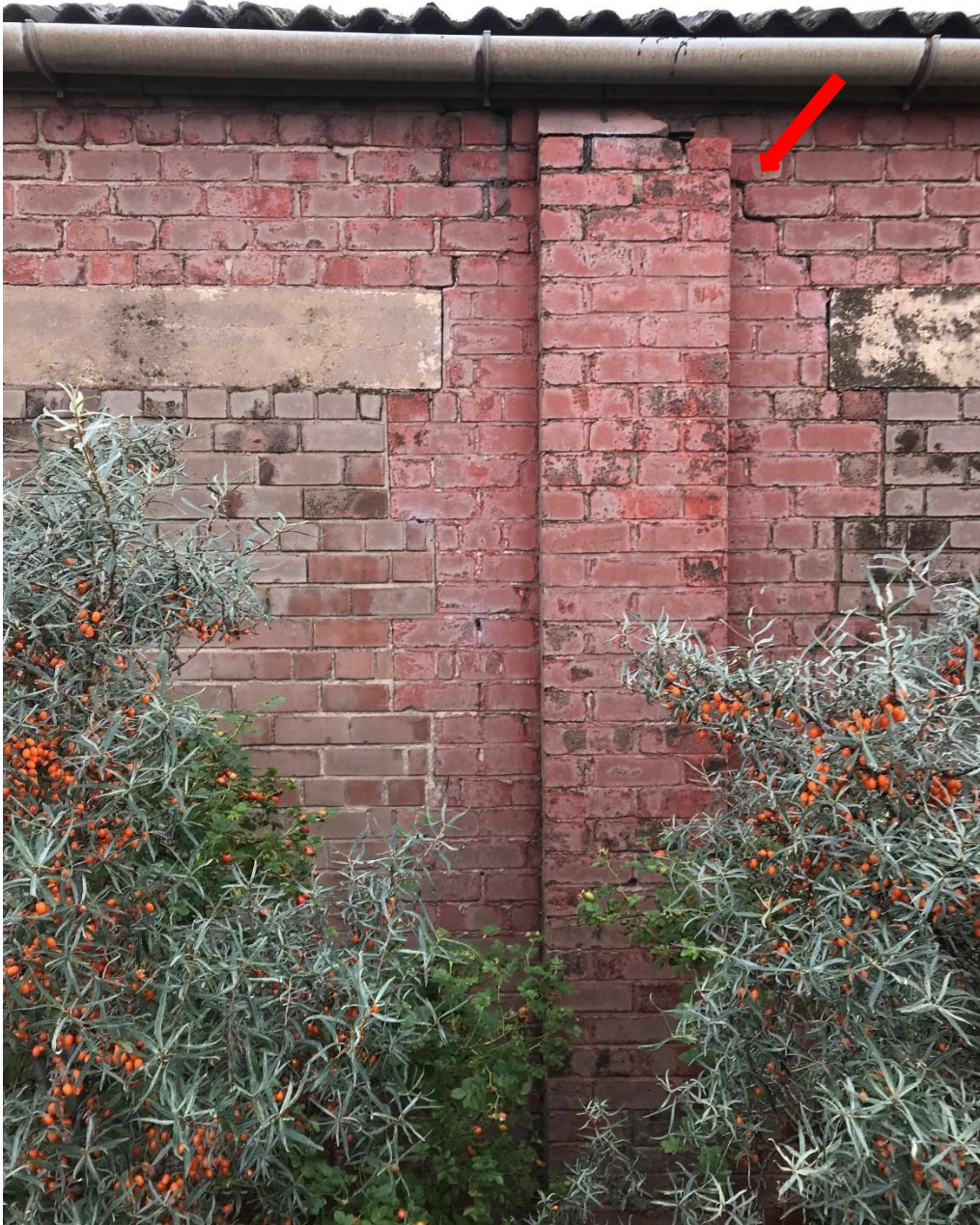
Photograph 9 – Gaps in mortar below fascia boarding, may lead to wall cavity of structure B1b
