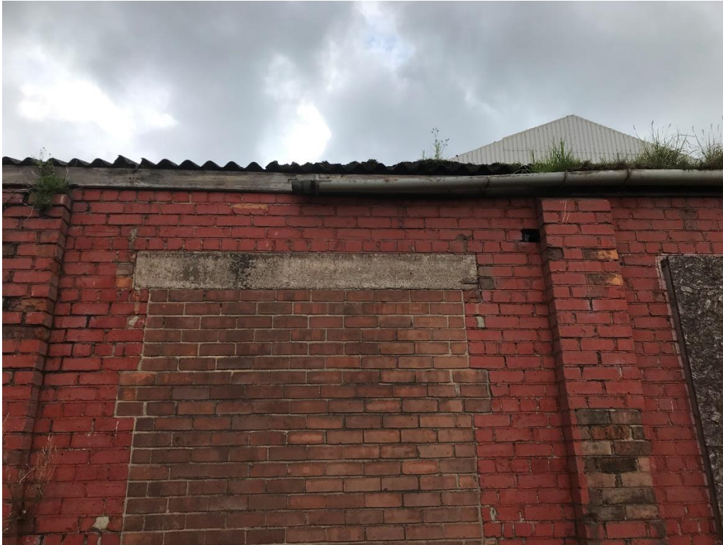
Photograph 7 – South-western aspect of structure B1b showing fascia boarding and failed guttering, mortar generally in good condition and fascia boarding fitted close against the wall
