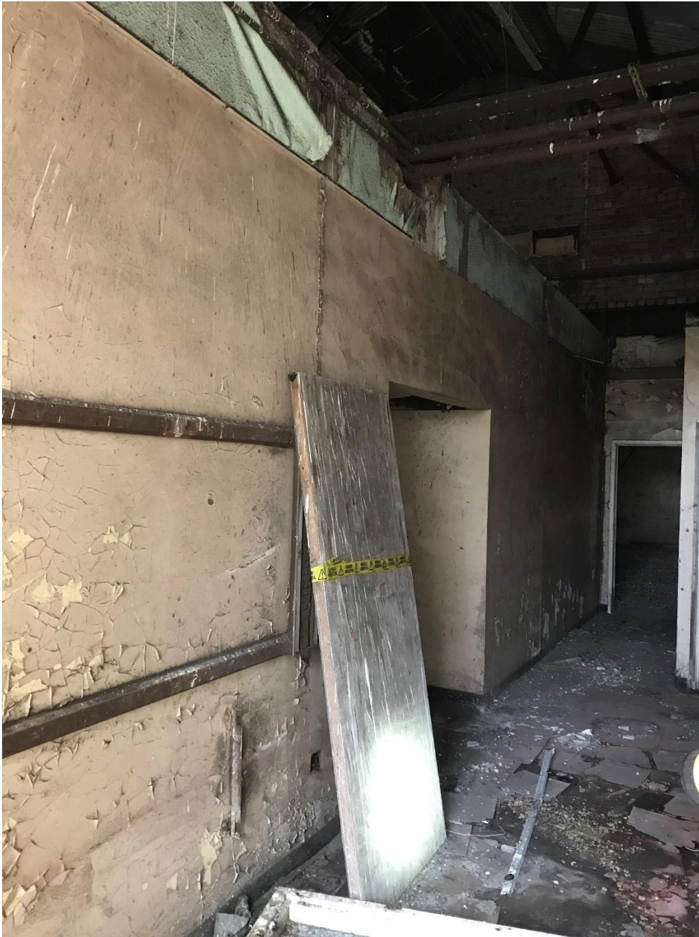
Photograph 11 – Interior of welfare block of structure B1b, showing rendered interior walls that stop well below roof height
