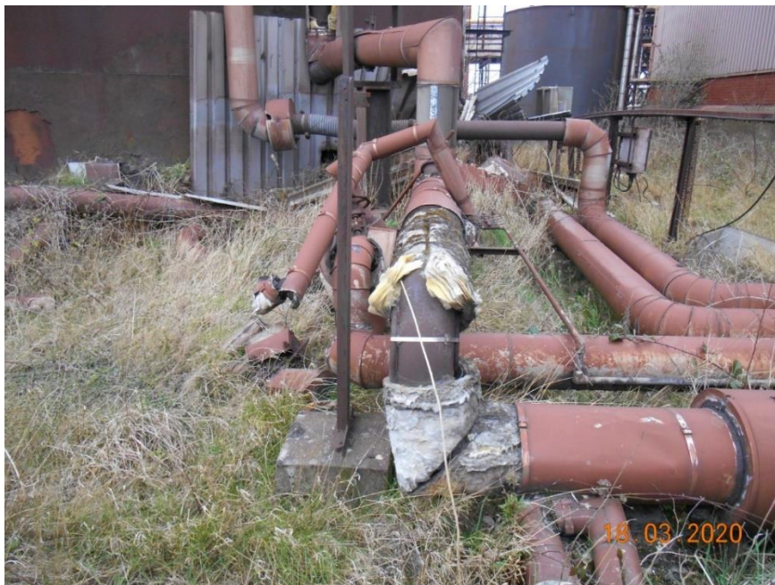
Plate 28 – Diesel tank connections and fibrous pipe lagging.
