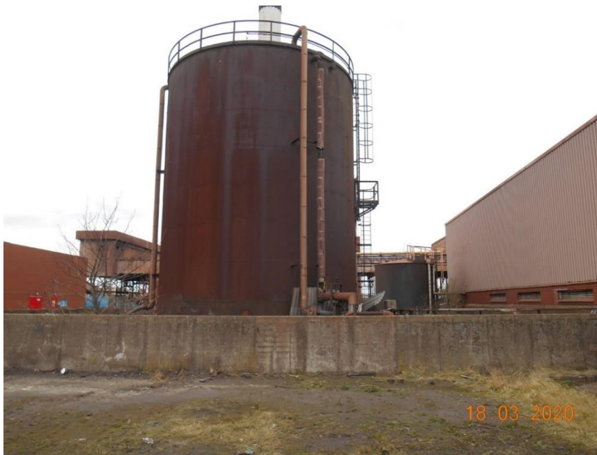
Plate 27 – View looking west northwest showing diesel tank and surrounding concrete bund wall.
