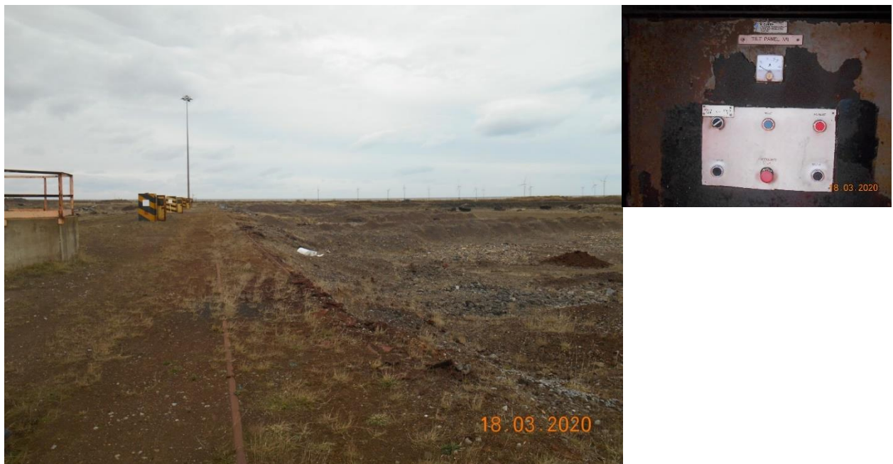
Plate 7 – View looking north west along the alignment of the steel torpedo 'pond area'. The tilt operation booths are seen yellow/black on the left hand side of the photograph (see insert showing Tilt Panel to the right), with running rails for the tippers shown on the edge of the 'pond' areas.
