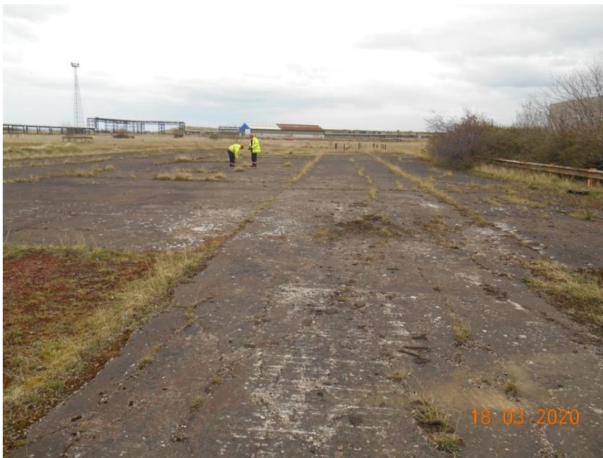
Plate 24 – View looking east southeast showing a hardstanding area. It was noted that the hardstanding surface is ‘wavy’ and cracked, again providing
