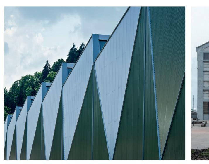
Cladding might be arranged in an Simple pitched roof forms angular format to create texture and interest. North facing rooflights allow natural light to penetrate the plant and limit the requirement for artificial lighting.
