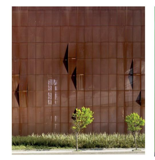
Mesh cladding would allow views through to the plant inside, using Cor-Ten steel would reflect the previous steelworks on the site. Hues of green mesh or cladding could be added, influenced by the surrounding landscape and would provide contrast with the rusty rich brown of the Cor-Ten.
